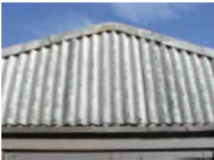
Asbestos cement wall panel
