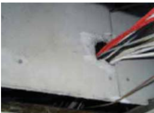
Asbestos insulating board panels
