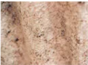
Sprayed coatings on ceiling, walls, beams/columns
