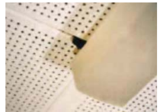
Asbestos insulating board ceiling tiles
