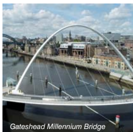
Gateshead Millennium Bridge
